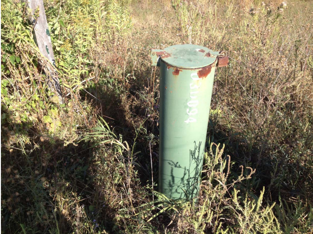
Site G, Monitoring Well 03U094 (uncertain of well ID – ID is worn). Well may need to be abandoned.
